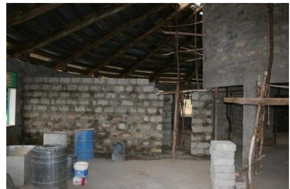
We are now focusing on completing the roof. We are also completing the inside walls. And we have started installing the electrical conduits.
